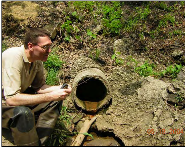
Figure 12: Dry weather field inspection
