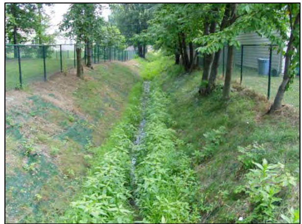
Figure 3: Ditch MS4 outfall
