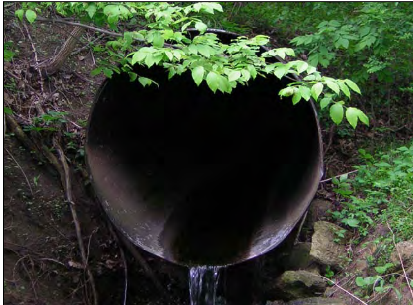
Figure 11: MS4 outfall location with illicit discharge
